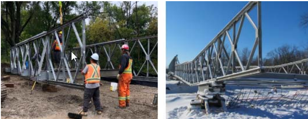
Figures 8 & 9: Assembly and Installation
