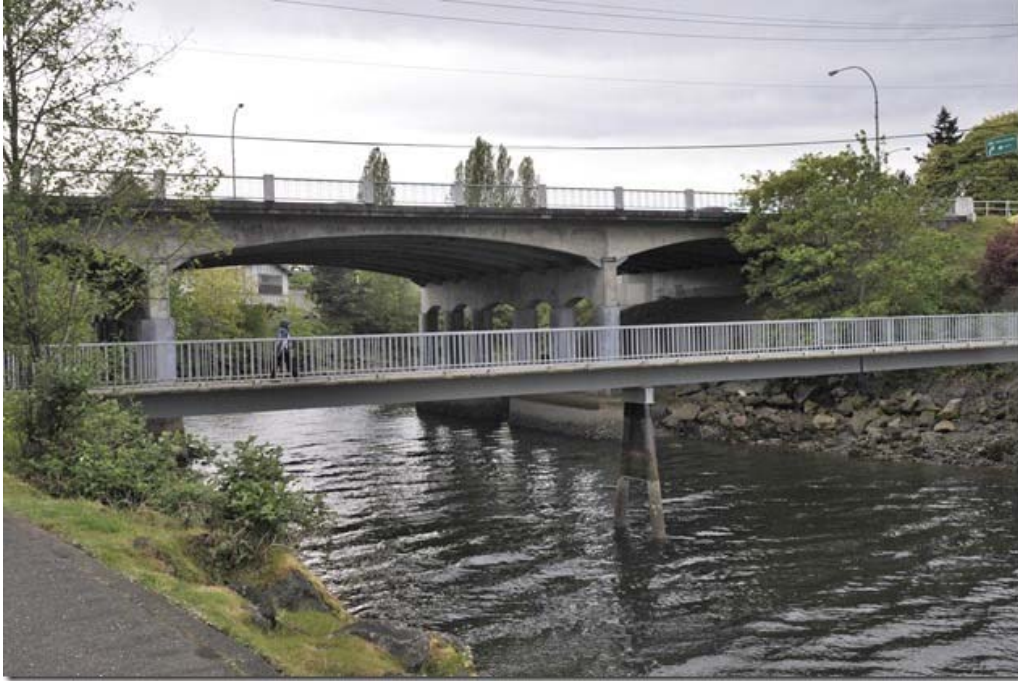
Figure 4: The active transportation bridge in Maffeo Sutton Park, Nanaimo, B.C.
