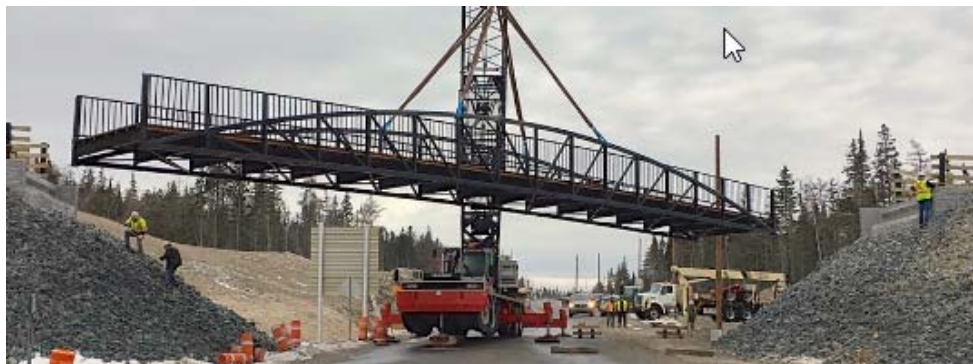
Figure 6: Installation of a Bowstring Truss Bridge
