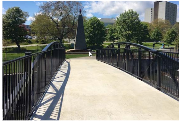
Figure 18: Bowstring Bridge Railing
