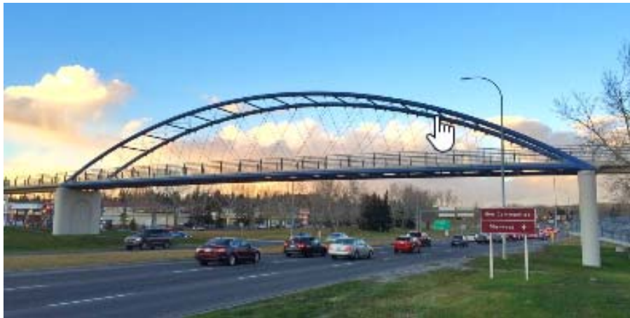
Figure 10: Network Arch Pedestrian Bridge Example
