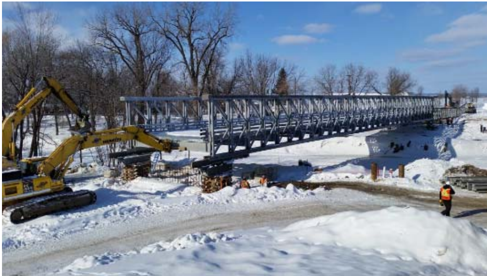
Figure 7: Modular Panel Bridge
